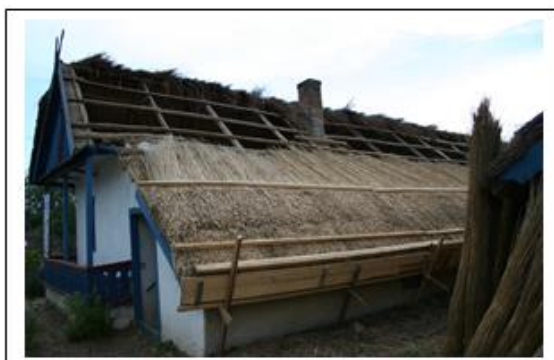
Photo 3. Rush cover. Stage of execution
